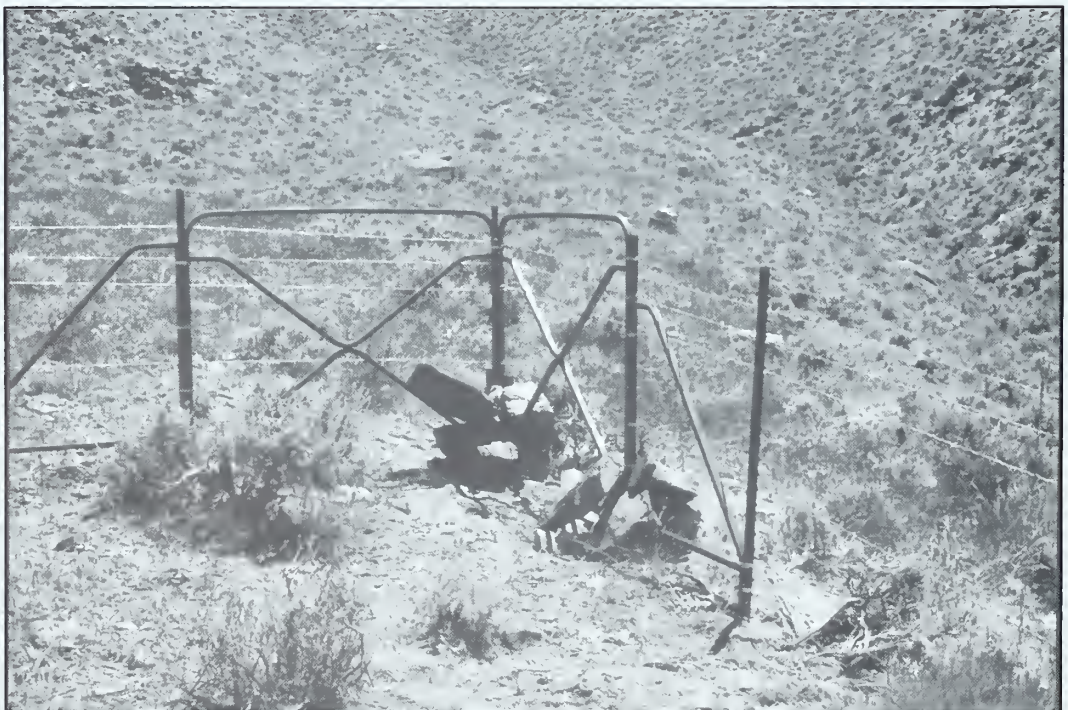
Photo 12. Barbed and smooth wire (bottom strand only) using steel "T" posts and "EZ" panel corners. Rocks (piled or wired on) strengthen the corner.
